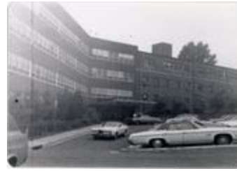
National Orthopaedic and Rehabilitation Hospital (21-5612)
