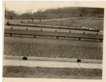
Water pollution control plant, 1940 (21-5372)
