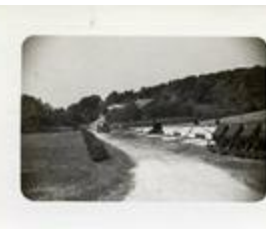
Sewage disposal plant sludge drying beds, 1942 (21-5492)
