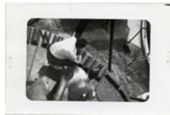
Sewage disposal plant sludge digestion tank, 1942 (21-5487)
