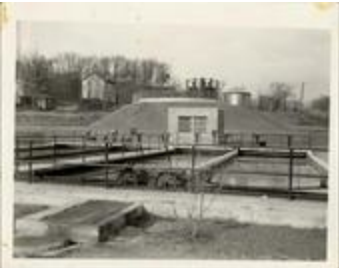
Water pollution control plant, 1940 (21-5371)
