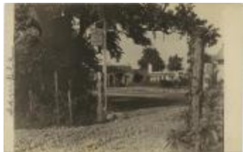
The Little Tea House Exterior with Signage (215-0035)
