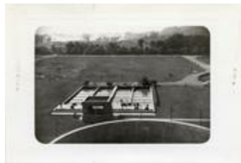
Sewage treatment plant primary settling tanks, 1942 (21-5483)
