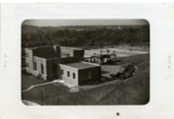
Sewage disposal plant and sludge beds, 1942 (21-5479)
