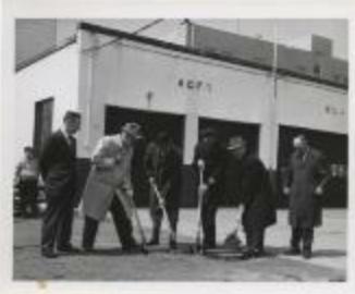
Fire Station #4 Groundbreaking (100-01-03-0238)
