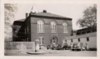
Arlington County Courthouse (100-03-01-0416)
