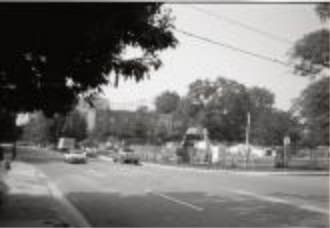
Construction on Quincy Street (250-05-01-3554)
