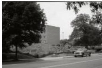
Demolition of 1110 and 116 Quincy Street (250-05-01-3542)
