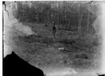
Construction Worker on Jewett Home Lot (123-02-06-0072)
