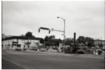
Construction of Eckerd Pharmacy (250-09-01-8772)
