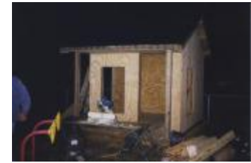
Construction at Night (332-05-08-0133)
