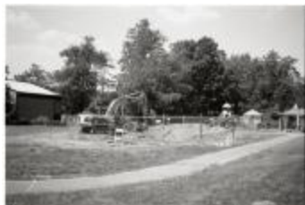
Fixing Water Main at Woodmont (250-05-01-3541)
