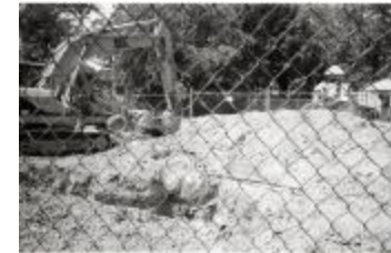
Fixing Water Main at Woodmont (250-05-01-3540)
