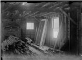
Interior of the Jewett Home Under Construction (123-02-06-0078)
