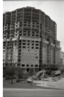
Construction of Arlington Courthouse Place (250-03-01-2884)
