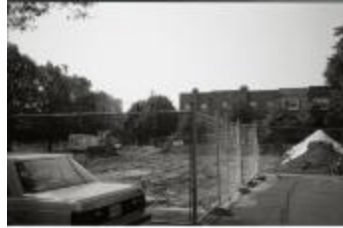
Construction on Quincy Street (250-05-01-3555)
