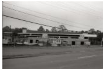
Construction of Barcroft Sports & Fitness Center (250-09-01-8770)
