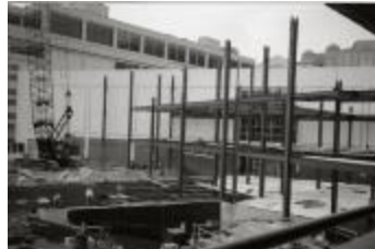
Hecht Company Office Tower Construction (250-05-01-3548)
