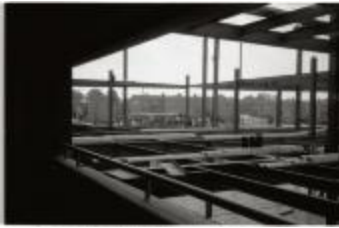
Hecht Company Office Tower Construction (250-05-01-3547)
