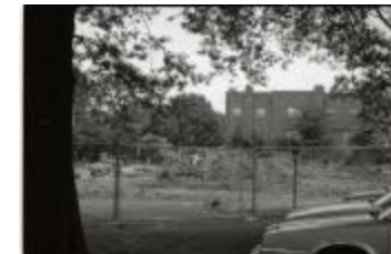
Demolition of 1110 and 116 Quincy Street (250-05-01-3544)
