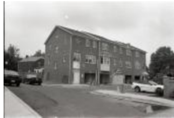
Construction of Arlington Heights Townes (250-09-01-8773)
