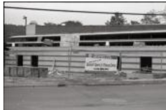
Construction of Barcroft Sports & Fitness Center (250-09-01-8769)
