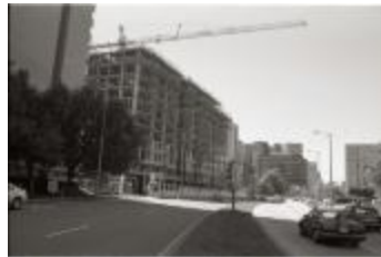
Construction on Fairfax Drive (250-09-01-8791)
