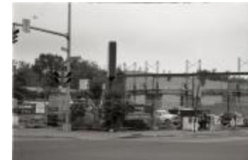
Construction of Eckerd Pharmacy (250-09-01-8771)
