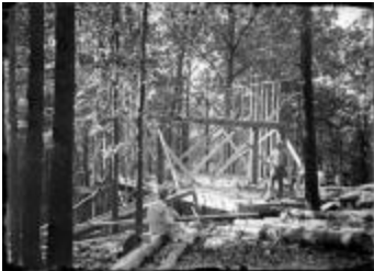
Frame of the Jewett Home Under Construction (123-02-06-0070)
