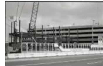
Hecht Company Office Tower Construction (250-05-01-3551)
