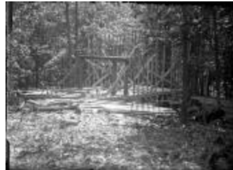
Frame of the Jewett Home Under Construction (123-02-06-0068)
