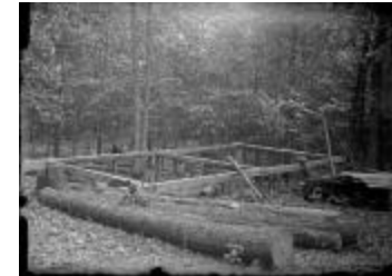
Early Frame of the Jewett Home Under Construction (123-02-06-0069)
