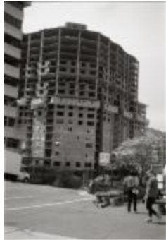
Construction of Arlington Courthouse Place (250-03-01-2883)
