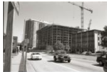
Construction on Fairfax Drive (250-09-01-8792)
