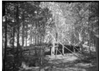
Frame of the Jewett Home Under Construction (123-02-06-0071)
