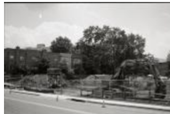
Demolition of 1110 and 116 Quincy Street (250-05-01-3543)
