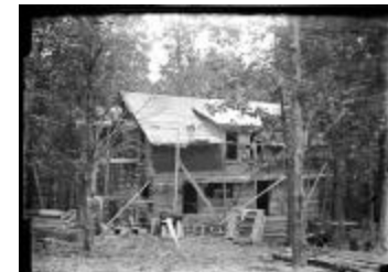
The Jewett Home Under Construction (123-02-06-0077)
