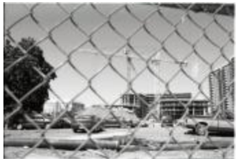
Construction on Wilson (250-09-01-8788)
