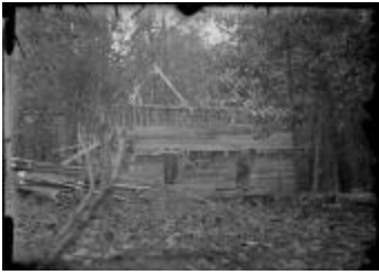
The Jewett Home Under Construction (123-02-06-0066)
