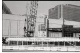
Hecht Company Office Tower Construction (250-05-01-3550)
