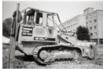
Dominion Front Loader on Site (250-05-01-3558)
