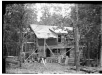
The Jewett Home Under Construction (123-02-06-0077)
