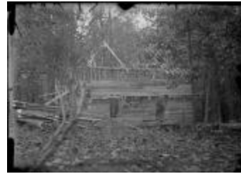
The Jewett Home Under Construction (123-02-06-0066)
