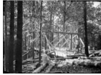
Frame of the Jewett Home Under Construction (123-02-06-0070)
