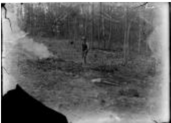
Construction Worker on Jewett Home Lot (123-02-06-0072)
