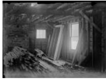
Interior of the Jewett Home Under Construction (123-02-06-0078)
