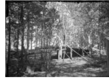
Frame of the Jewett Home Under Construction (123-02-06-0071)
