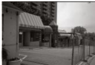
Closed Strip Mall on Courthouse Road (250-03-01-2876)
