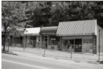
Closed Strip Mall on Courthouse Road (250-03-01-2879)
