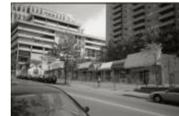
Closed Strip Mall on Courthouse Road (250-03-01-2878)
