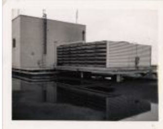
Air Conditioning Tower on the Courthouse Roof (100-03-01-0406)
