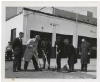
Fire Station #4 Groundbreaking (100-01-03-0238)
