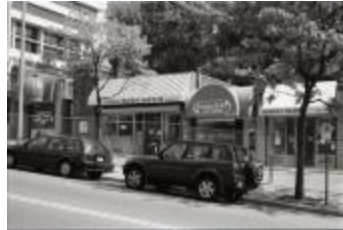
Closed Strip Mall on Courthouse Road (250-03-01-2880)
