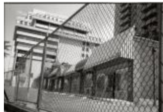
Closed Strip Mall on Courthouse Road (250-03-01-2877)
