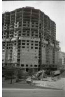
Construction of Arlington Courthouse Place (250-03-01-2884)
