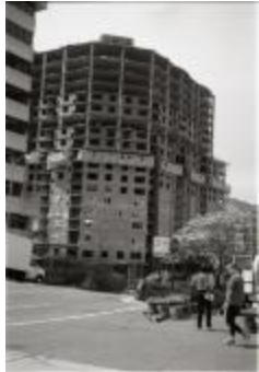
Construction of Arlington Courthouse Place (250-03-01-2883)
