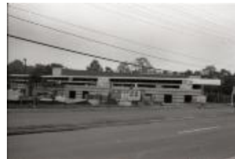
Construction of Barcroft Sports & Fitness Center (250-09-01-8770)
