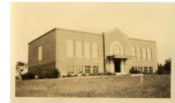
Barcroft School Building (32-07-08-01-0135)
