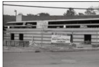
Construction of Barcroft Sports & Fitness Center (250-09-01-8769)
