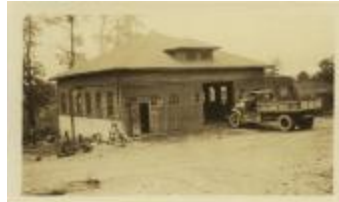
Farm Repair Shop (32-07-08-02-0167)
