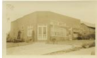
Virginia Highlands Health Center (32-07-08-02-0171)
