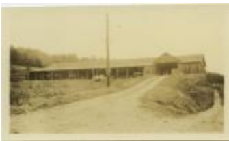
Farm Main Barn (32-07-08-02-0163)
