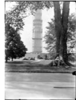
Washington Monument Under Construction (123-02-16-0048)
