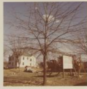
Central Library Construction Site (29-01-13-01-0062)
