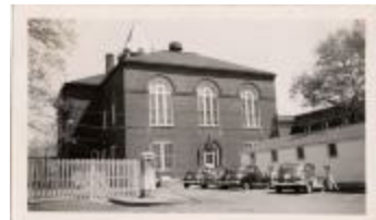
Arlington County Courthouse (100-03-01-0416)
