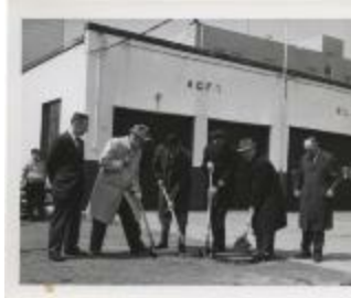
Fire Station #4 Groundbreaking (100-01-03-0238)
