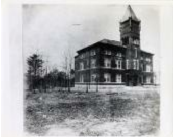
Arlington County Courthouse (100-03-01-0402)
