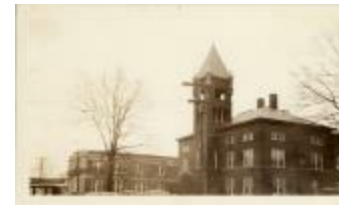
Arlington County Courthouse (100-03-01-0401)
