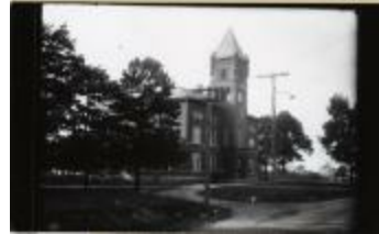
Arlington County Courthouse (100-03-01-0403)
