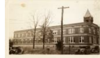
Arlington County Courthouse (100-03-01-0405)
