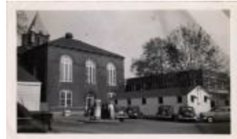
Arlington County Courthouse (100-03-01-0408)
