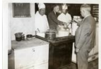
Evans Coffee Shop Kitchen Inspection (21-5232)
