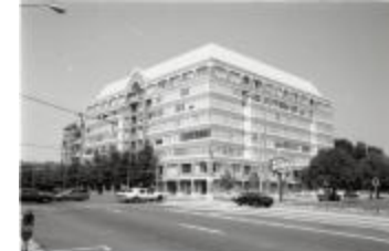
Quincy Street Station (250-06-01-3606)
