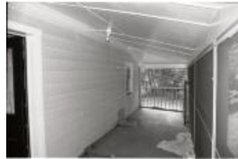
Upstairs Porch Outside Basil Hall House (250-08-01-8763)
