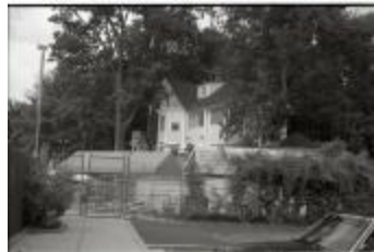
Febrey-Kincheloe House, from parking lot, 1997 (250-01-01-1306)
