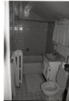
Basil Hall House Bathroom (250-08-01-8761)
