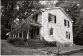
Side and Porch of Basil Hall House (250-08-01-8750)
