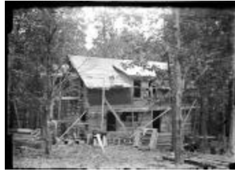
The Jewett Home Under Construction (123-02-06-0077)
