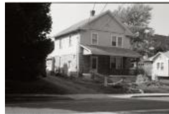
1110 and 1116 Quincy Street North (250-02-01-1323)
