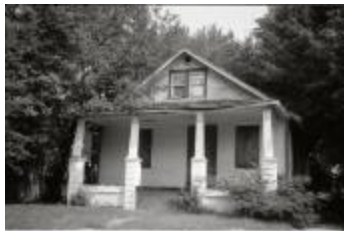
4007 11th Street North (250-05-01-3556)
