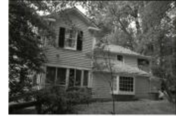
Side of Basil Hall House (250-08-01-8749)
