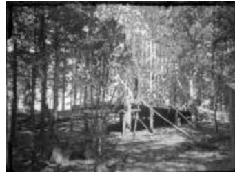
Frame of the Jewett Home Under Construction (123-02-06-0071)
