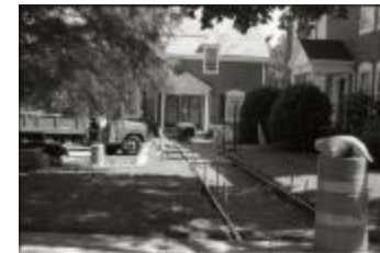
New Sidewalks at Fairlington Commons (250-09-01-8781)
