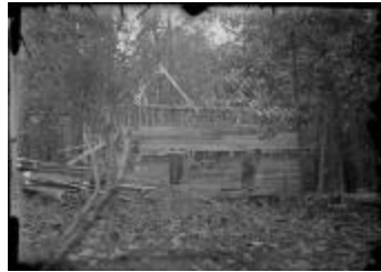
The Jewett Home Under Construction (123-02-06-0066)
