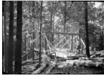
Frame of the Jewett Home Under Construction (123-02-06-0070)
