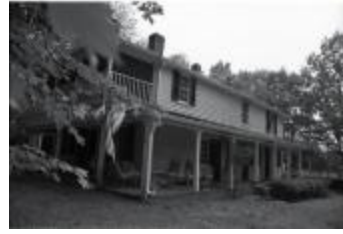
Basil Hall House Front Porch (250-08-01-8747)
