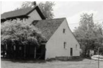
Ball-Sellers House, Original Structure, 1996 (202-6240)
