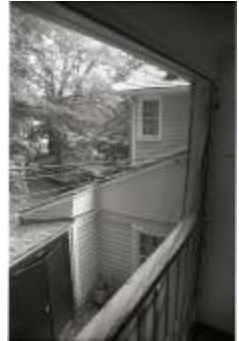
View from Upstairs Porch at Basil Hall House (250-08-01-8762)
