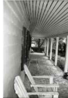
Basil Hall House Front Porch (250-08-01-8766)
