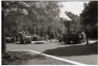
New Sidewalks at Fairlington Commons (250-09-01-8782)
