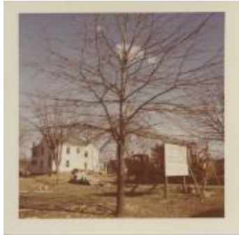
Central Library Construction Site (29-01-13- 01-0062)
