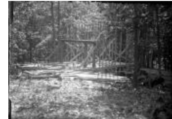
Frame of the Jewett Home Under Construction (123-02-06-0068)
