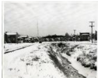
Open Drain in Snow (32-07-07-17-0133)
