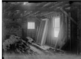
Interior of the Jewett Home Under Construction (123-02-06-0078)
