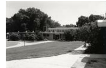
Tuckahoe Elementary School, 2006 (202-6178)
