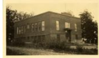
Kemper School Building (32-07-08-01-0146)
