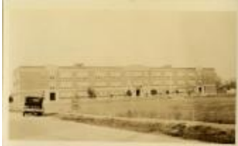
Washington-Lee School Building (32-07-08-01-0154)
