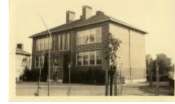
New Cherrydale School Building (32-07-08-01-0137)
