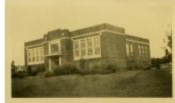
Henry Clay School Building (32-07-08-01-0139)
