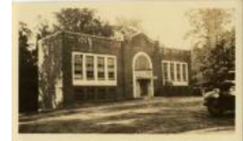
Woodmont School Building (32-07-08-01-0156)
