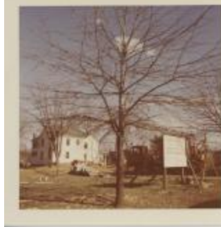
Central Library Construction Site (29-01-13-01-0062)
