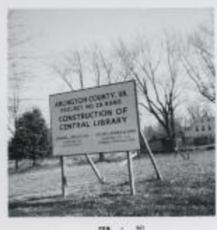
Arlington Central Library Construction (29-01-13-01-0058)
