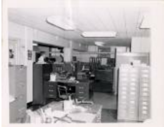
Courthouse Basement, South Wing, IBM section (100-03-01-0425)
