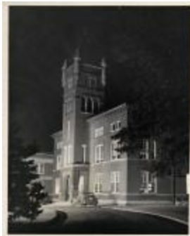
County Courthouse at Night (100-03-01-0420)
