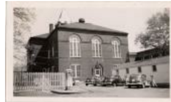
Arlington County Courthouse (100-03-01-0416)
