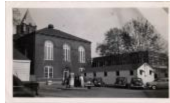
Arlington County Courthouse (100-03-01-0408)
