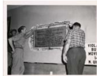
Plaque in the Old Courthouse Lobby (100-03-01-0422)
