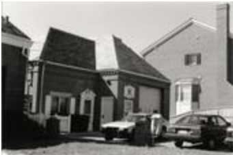
Arlington County Fire Station 7 Fairlington, 1996 (202-6146)
