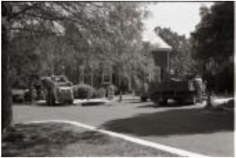
New Sidewalks at Fairlington Commons (250-09-01-8782)
