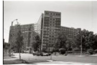
Riverhouse Apartment Building (250-09-01-8785)
