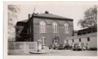
Arlington County Courthouse (100-03-01-0416)
