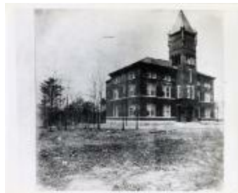
Arlington County Courthouse (100-03-01-0402)
