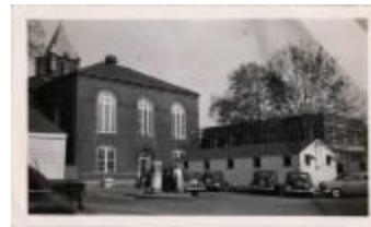
Arlington County Courthouse (100-03-01-0408)
