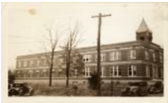
Arlington County Courthouse (100-03-01-0405)
