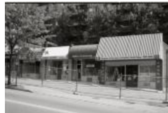
Closed Strip Mall on Courthouse Road (250-03-01-2879)
