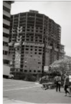
Construction of Arlington Courthouse Place (250-03-01-2883)
