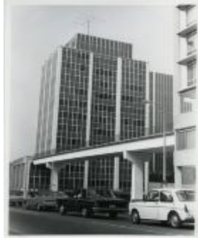
Rosslyn Pedestrian Bridge (214-03-01-9314)
