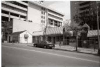
Closed Strip Mall on Courthouse Road (250-03-01-2881)
