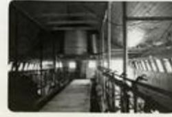
Interior of Barn at Rose Hill Farm Dairy, 1942 (21-5513)
