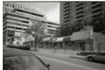
Closed Strip Mall on Courthouse Road (250-03-01-2878)
