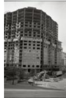
Construction of Arlington Courthouse Place (250-03-01-2884)
