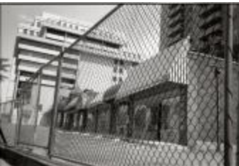
Closed Strip Mall on Courthouse Road (250-03-01-2877)
