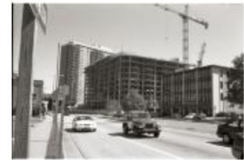
Construction on Fairfax Drive (250-09-01-8792)
