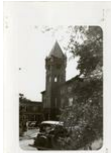
Arlington County Courthouse, 1942 (21-5474)
