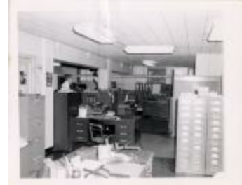
Courthouse Basement, South Wing, IBM section (100-03-01-0425)
