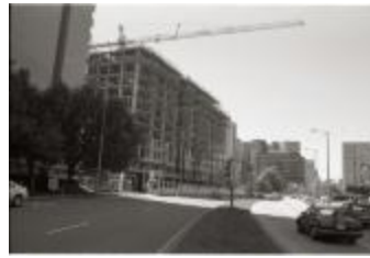
Construction on Fairfax Drive (250-09-01-8791)
