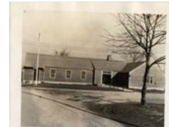
Defense Housing Administration Building, 1943 (21-5315)
