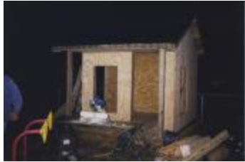
Construction at Night (332-05-08-0133)
