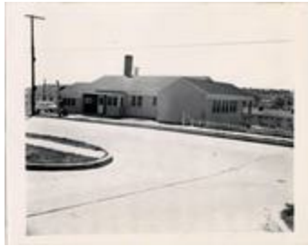
Dunbar Health Center, 3500 South Kemper Road, 1958 (21-5442)
