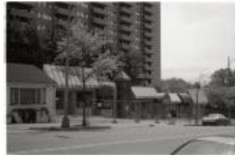
Closed Strip Mall on Courthouse Road (250-03-01-2882)
