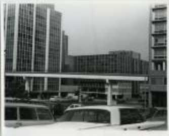
Rosslyn Pedestrian Bridge (214-03-01-9313)
