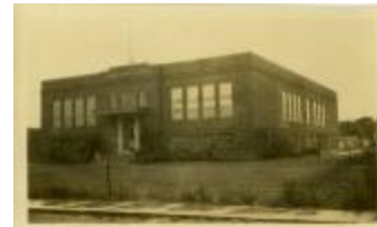
James Monroe School Building (32-07-08-01-0141)
