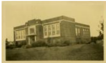
Henry Clay School Building (32-07-08-01-0139)
