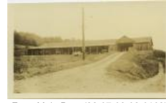
Farm Main Barn (32-07-08-02-0163)
