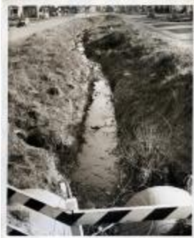
Culvert and Open Drain (32-07-07-17-0131)
