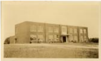
Jefferson Colored School, Main Building (32-07-08-01-0143)
