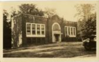
Woodmont School Building (32-07-08-01-0156)
