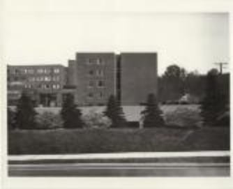
Hospital From Street, Garage (32-04-11-12-0120)
