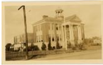
Woodrow Wilson School Building (32-07-08-01-0157)
