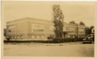
Nellie Custis School Building (32-07-08-01-0148)
