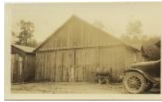
Old Blacksmith Shop (32-07-08-02-0166)
