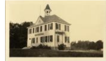
Saegmuller School Building (32-07-08-01-0151)
