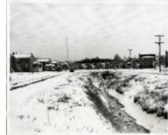
Open Drain in Snow (32-07-07-17-0133)
