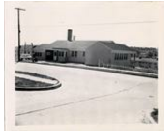
Dunbar Health Center, 3500 South Kemper Road, 1958 (21-5442)
