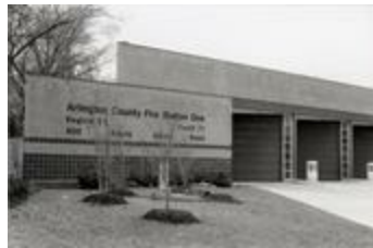
Arlington County Fire Station 1 Glebe Road, 1996 (202-6138)
