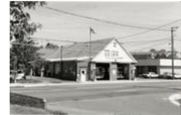
Arlington County Fire Station 6 Falls Church, 1996 (202-6145)
