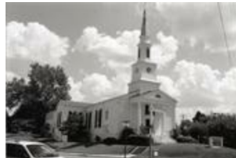
Walker Chapel United Methodist Church, 1996 (202-6121)
