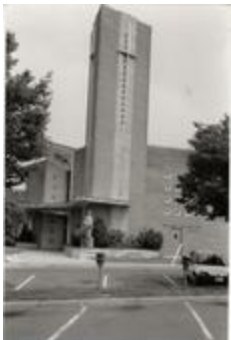
St. Charles Borromeo Catholic Church, 1996 (202-6101)
