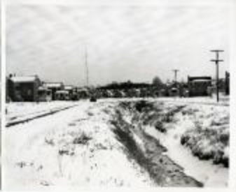
Open Drain in Snow (32-07-07-17-0133)
