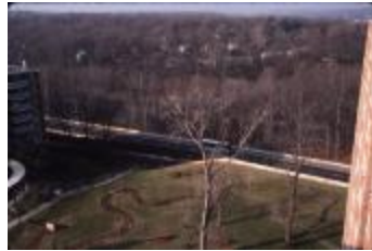
Completed I-66 from Above (210-0006)
