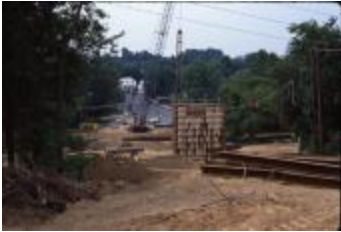
Construction of the Patrick Henry Overpass and I-66 (210-0017)
