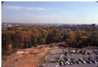
Construction Area of I-66 from Above (210-0009)
