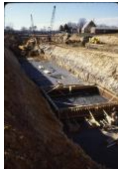
Pouring Concrete for I-66 (210-0045)
