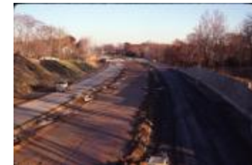
Construction of I-66 from the Patrick Henry Overpass (210-0047)
