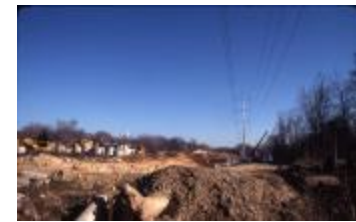
Construction of I-66 Near McKinley Road (210-0012)
