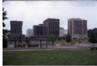
Rosslyn Circle Bus Terminal (210-0029)
