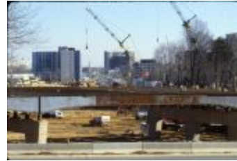
Construction of the George Mason Bridge (210-0042)
