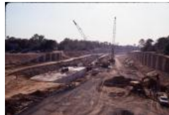
Construction of I-66 (210-0046)
