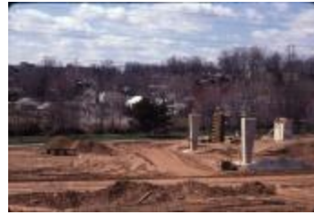
Construction of the Pedestrian Overpass at N. Potomac Street (210-0049)
