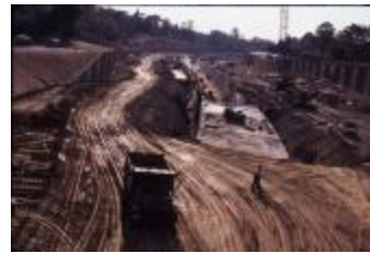
Construction of the Metro Surface Point on I-66 (210-0003)
