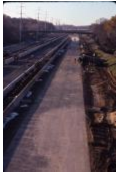
I-66 and Metro Construction (210-0048)
