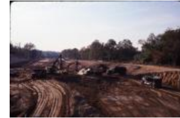
Construction of I-66 (210-0043)
