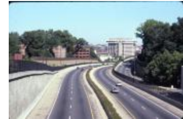
Completed Section of I-66 Going Through Rosslyn (210-0016)
