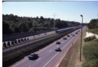
Completed I-66 from the Patrick Henry Overpass (210-0015)
