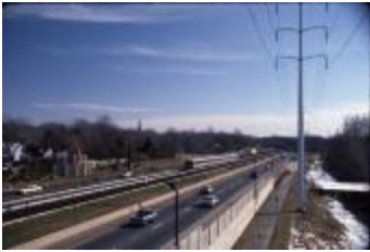
Completed I-66 Near Westover Baptist (210-0013)
