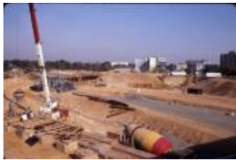
Construction of I-66 in Ballston (210-0001)
