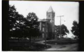
Arlington County Courthouse (100-03-01-0403)
