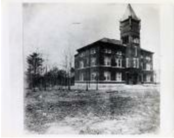
Arlington County Courthouse (100-03-01-0402)
