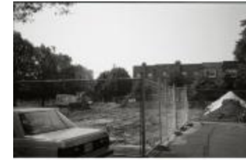
Construction on Quincy Street (250-05-01-3555)
