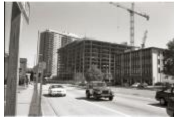
Construction on Fairfax Drive (250-09-01-8792)
