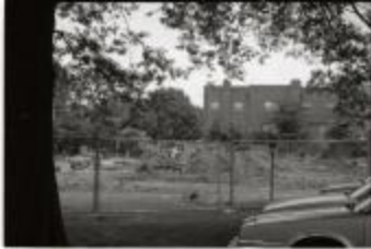
Demolition of 1110 and 116 Quincy Street (250-05-01-3544)
