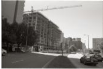
Construction on Fairfax Drive (250-09-01-8791)
