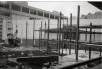
Hecht Company Office Tower Construction (250-05-01-3548)
