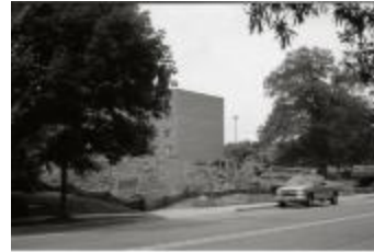
Demolition of 1110 and 116 Quincy Street (250-05-01-3542)
