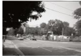
Construction on Quincy Street (250-05-01-3554)
