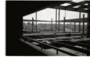
Hecht Company Office Tower Construction (250-05-01-3547)
