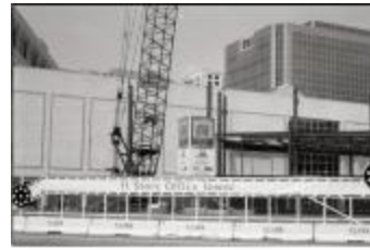
Hecht Company Office Tower Construction (250-05-01-3550)
