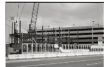
Hecht Company Office Tower Construction (250-05-01-3551)
