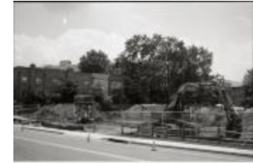
Demolition of 1110 and 116 Quincy Street (250-05-01-3543)
