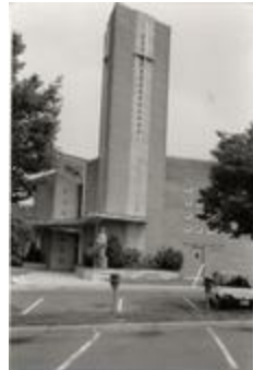
St. Charles Borromeo Catholic Church, 1996 (202-6101)
