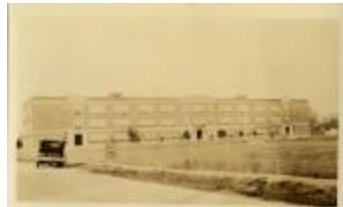
Washington-Lee School Building (32-07-08-01-0154)
