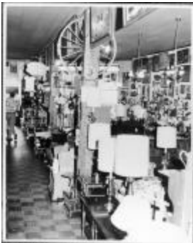
Columbia Furniture, Interior View (212-8730)
