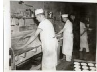
Inspection of Millers Bakery (21-5236)
