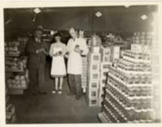
Inspection of Grocery Store, 1942 (21-5293)
