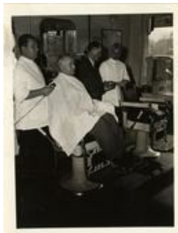
Inspection of Barber Shop, 1943 (21-5321)
