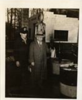
Inspection of Oil Tank, 1943 (21-5323)
